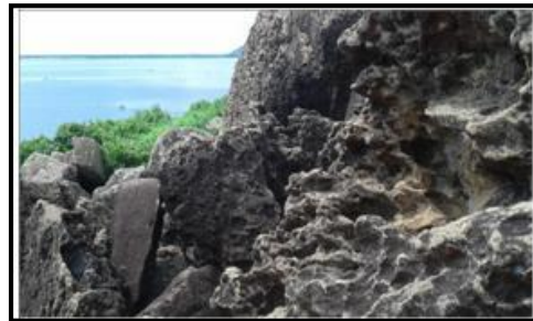
Fig 14 Solution Cavities in coastal rock (Photo courtesy Dr BM Faruque.)
